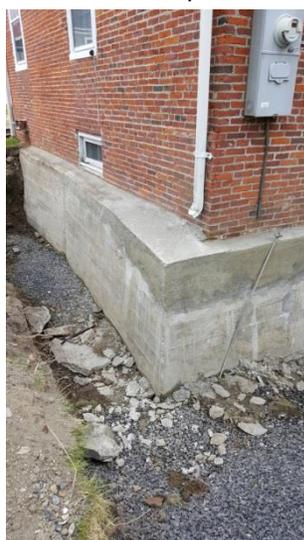
After preparing the drainage ditch for laying the eventual drainage pipes, the next step was sealing the foundation . . . which involved a
