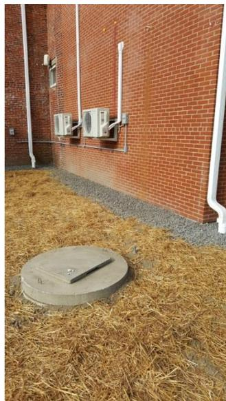
The water is pulled to a new drainage well with a powerful pump which sends water out from the drainage well through underground pipes we've laid under the driveway road out to the storm ditch on Thatcher Street.
